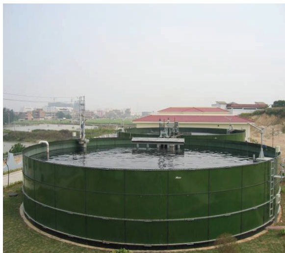
Fig. 7 Bolted two-coat enamel sediment tank –Industrial waste water treatment system in Quanzhou
