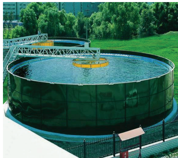
Fig. 6 Bolted two-coat enamel cyclone tank – sewage treatment system for Beijing Olympic Game 2008
