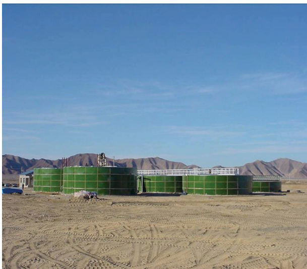
Fig. 5 Bolted two-coat enamel tank – water treatment system of Jiuquan Satellite Launching Center
