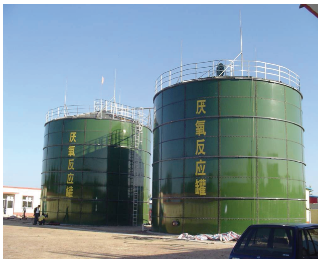
Fig. 8 Two-coat enamel anaerobic reaction vessel – biological power plant of Xisen Sanhe Group
