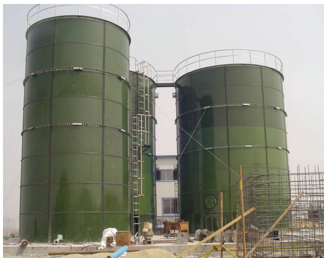
Fig. 10 Bolted two-coat enamel reactor in Tai'an Brewery
