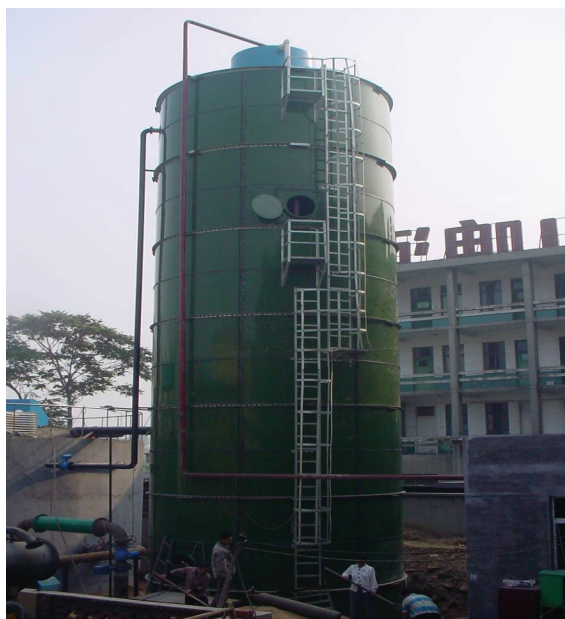
Fig. 9 Bolted two-coat enamel reactor or Garbage Disposal System in Jinjing
