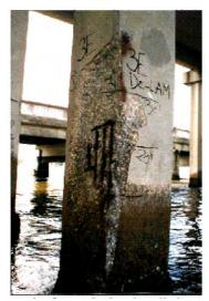
bond with the underlying steel and the water-rich paste immediately adjacent to the steel is typically weaker than the average paste in the mass of concrete.
